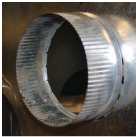
Figure 2: Install the 6" duct collar.
